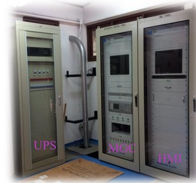
Microgrid Controller
